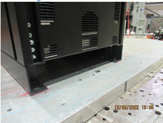
Figure 8: UUT1 Pre-Test Condition
