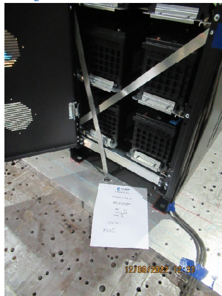
Figure 26: Run 2 Post-Test Condition
