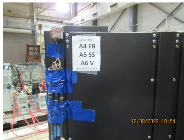
Figure 2: Placement of A4, A5, and A6
