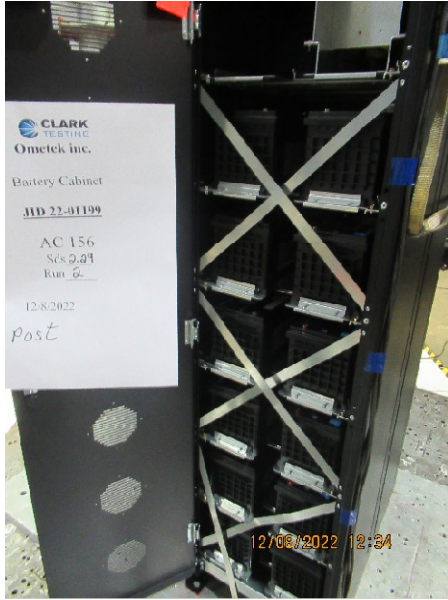
Figure 27: Run 2 Post-Test Condition
