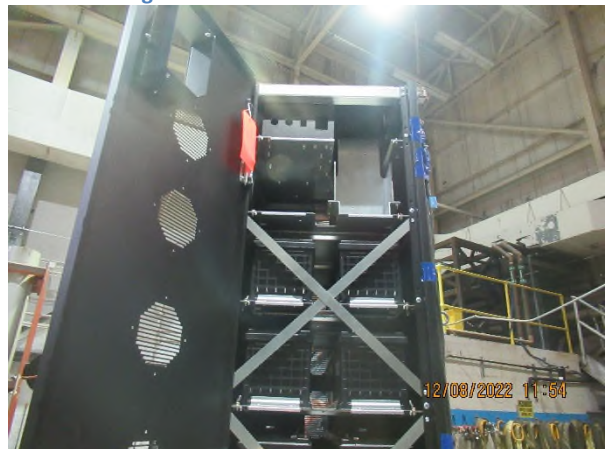
Figure 19: Run 1 Post-Test Condition
