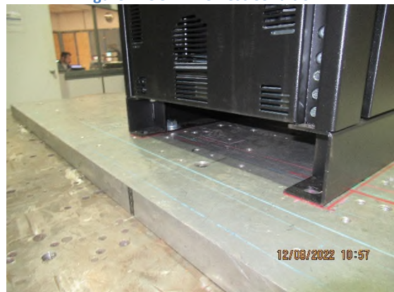
Figure 9: UUT1 Pre-Test Condition
