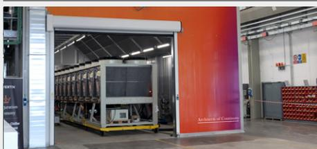
The Freecooling Chiller Validation Area is able to balance a thermal load of up to 1600 kW with a chamber air temperature between 20°C and 50°C and chiller water set point between 5°C and 20°C.
